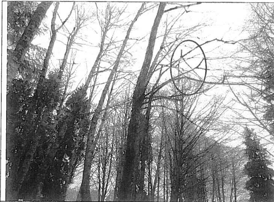
PHOTO 8: Note limb shedding hazards (red circle) at Stink Creek Park which will intensify as the Alder get larger. Attempt to space out the alder, removing defective stems, stems with crowns overlapping their neighbour, or to release understory conifers.
