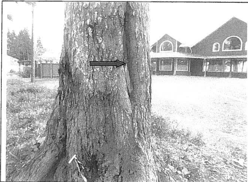
PHOTO 4: View of the damaged stem of tree #4862 which has advanced decay. In addition, this Hw tree's roots are also damaged and decaying, making it a high risk tree.
