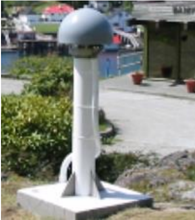
GNSS monument with GNSS antenna (receiver)
